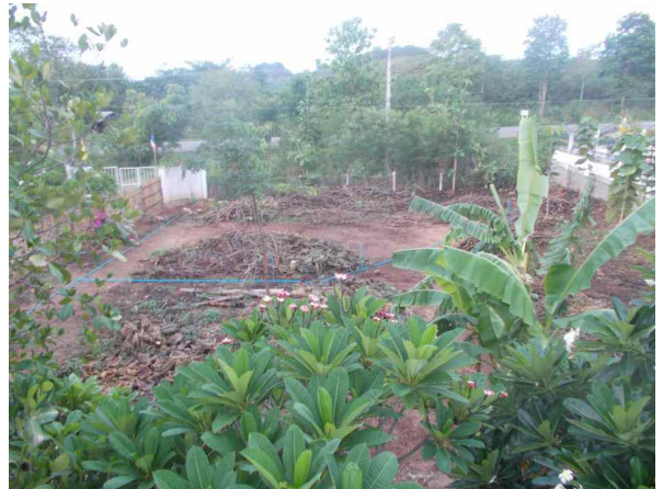
New water pipes (blue) in our garden
