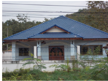
The house of Khun Suriya seen from the Highway 323
