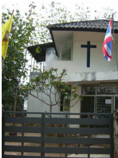
The new roof above our office
