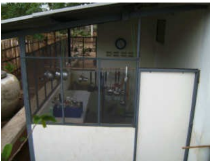
The new kitchen seen from outside
