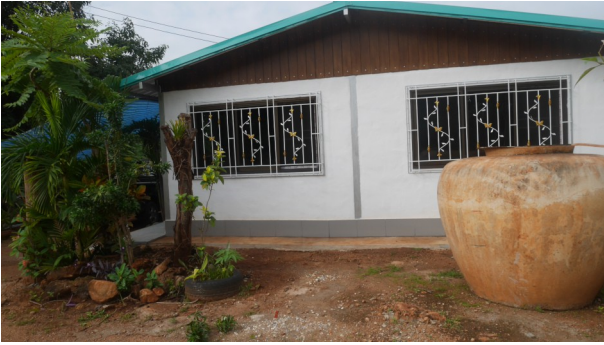
The office of our foundation is now ready.
