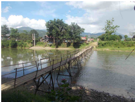
Vangvieng: Footbridge across the river
