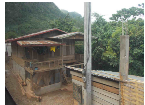
at a mountain pass: The right side of this house is supported by long beams.
