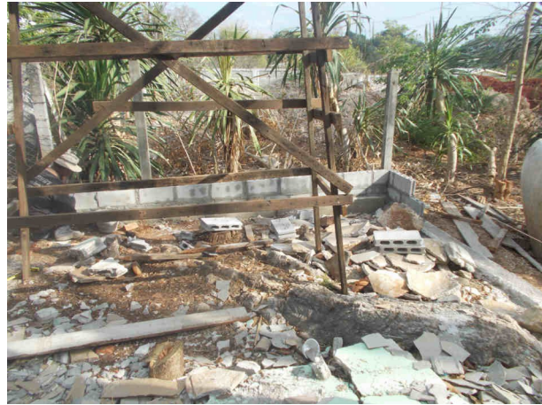
Here will be the rest room.
