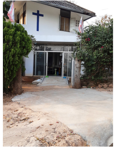
The ramp to house 2
