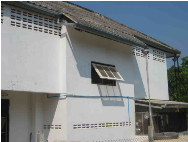
House 2: Here a bit of paint is yet lacking.
